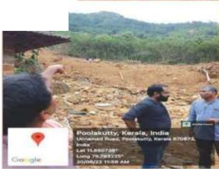
Landslide kanichar panchayath
